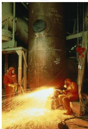
Figure 2: G2 Dismantling operation
