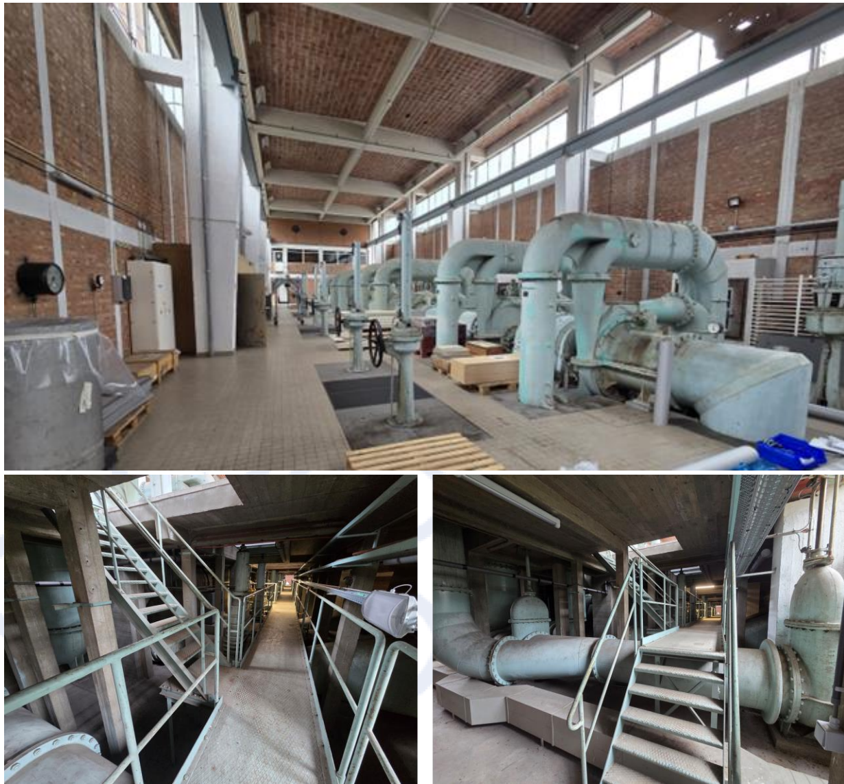
Figure 8: BR1 ventilation building. a) Large-volume area with engines and ventilators (top view); b) Dense infrastructure, such as piping, pumps and low-ceilings (bottom view)
